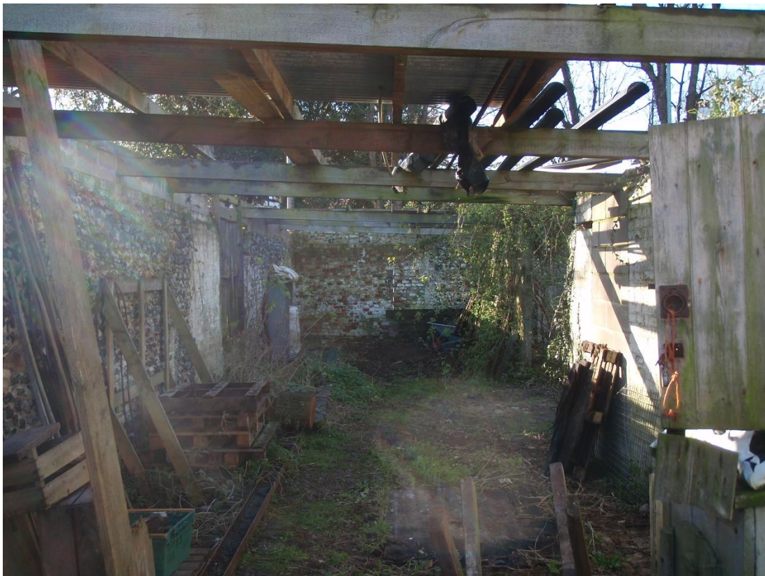
Plate 8. Internal view (looking south)
