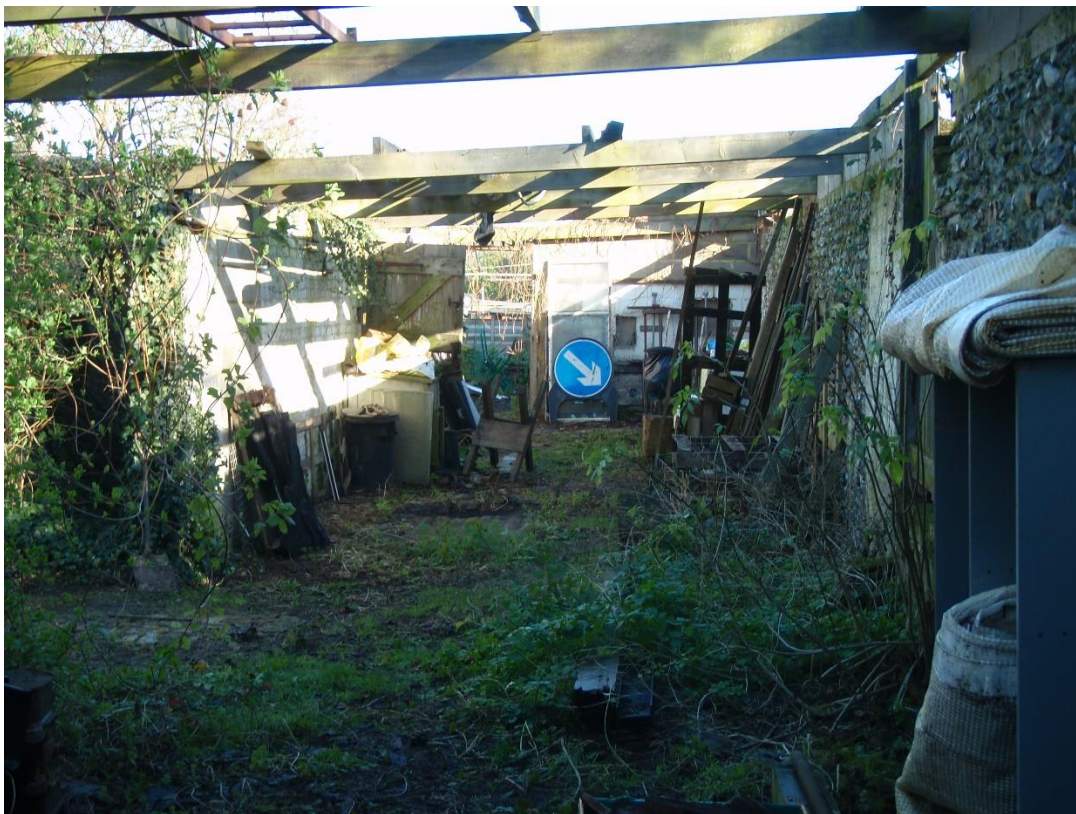
Plate 2. Interior (looking north)
