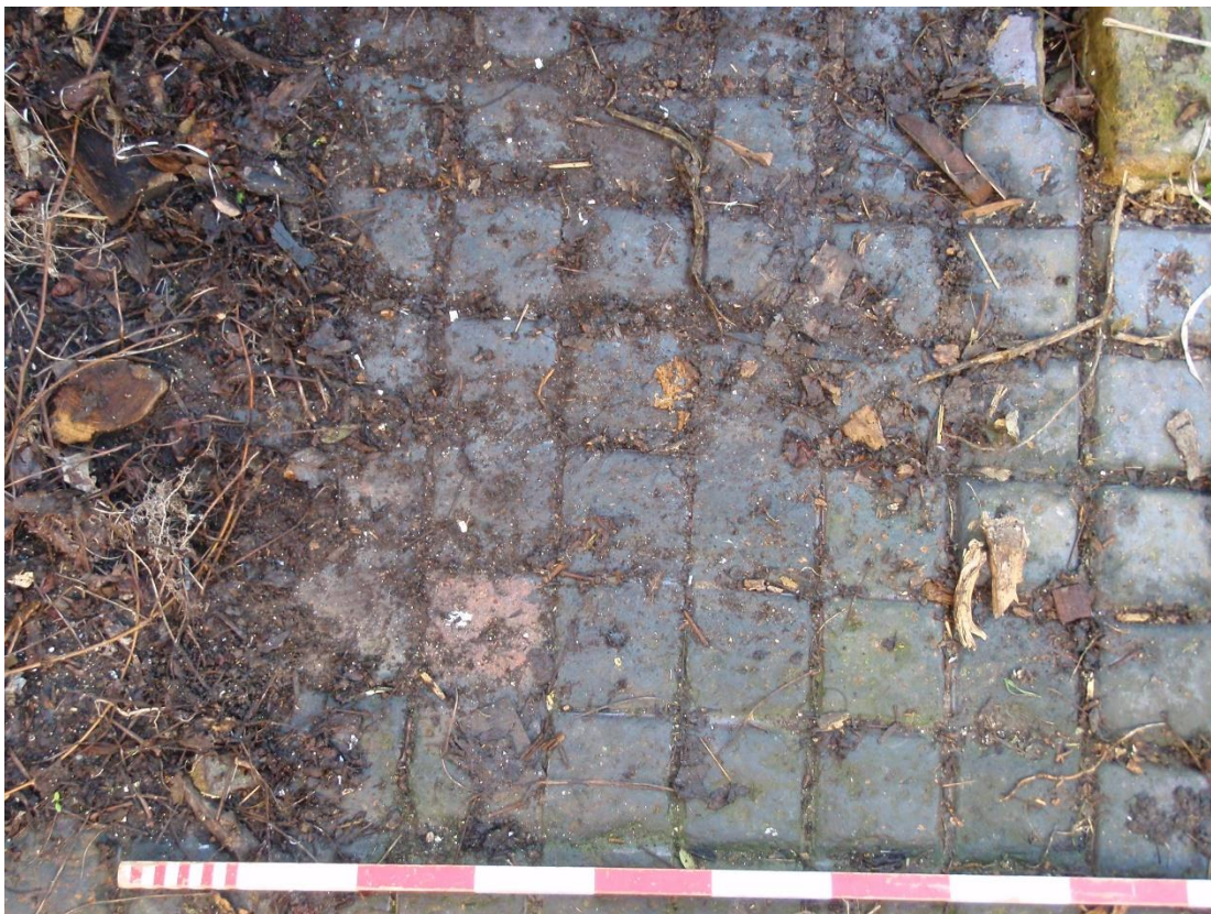
Plate 10. View of internal brick setts north end
