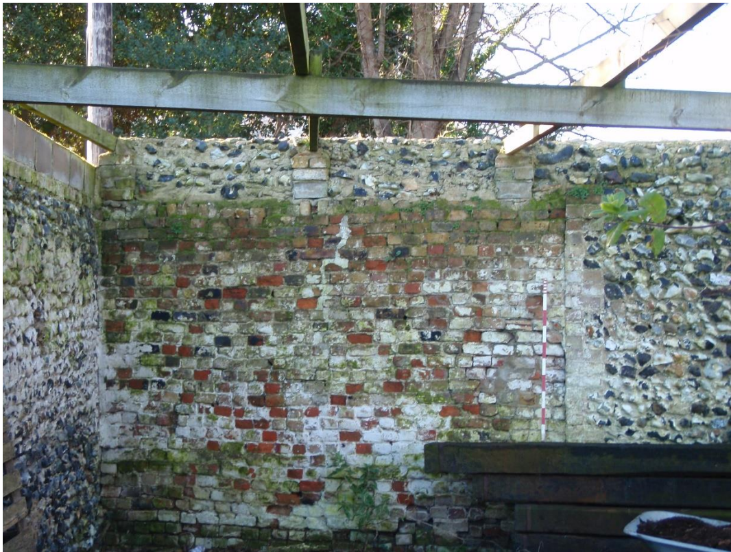
Plate 1. Internal south facing wall
