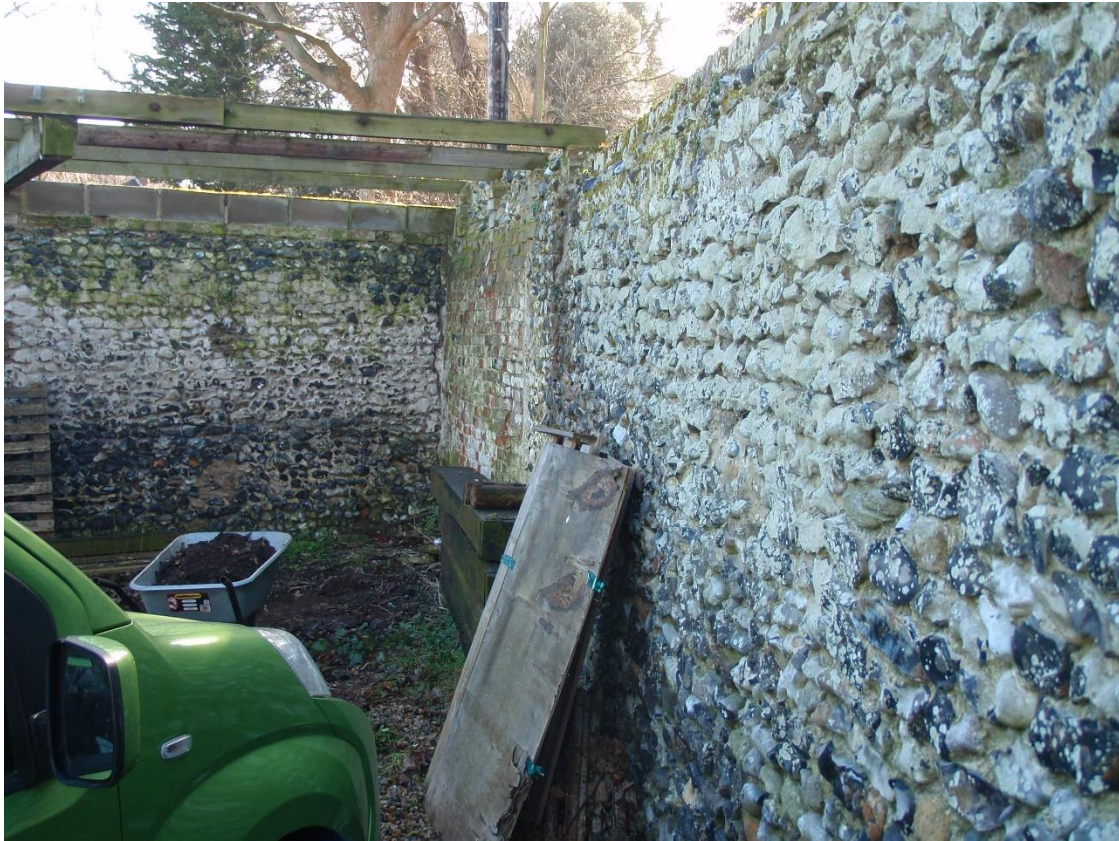
Plate 11. Internal view of north-west wall to be demolished
